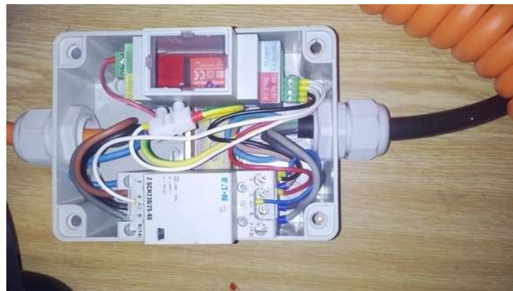
Picture 14: Charging cable made with EVSE DIN together with 4pole contactor in a box
